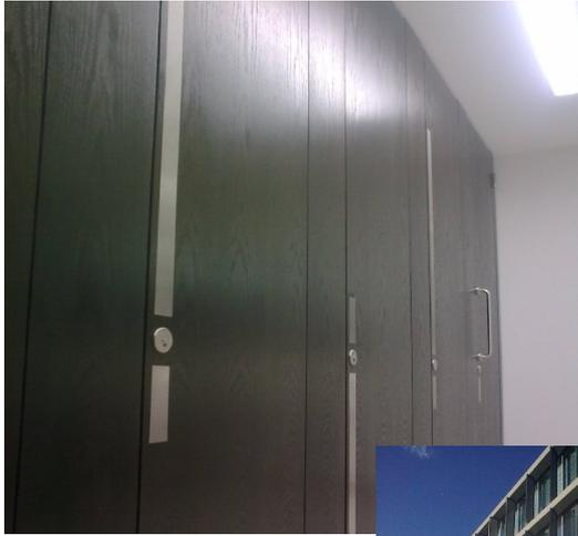
Working with Wates Construction, Shire were appointed as the washroom installer at the Jacobs Engineering project at Winnersh Triangle in Reading. The work involved the installation of a high end cubicle system as manufactured by Amwell Systems Ltd, called Sytan. This involved the design of a flush fronted veneered cubicle system, along with associated WC duct panels.
